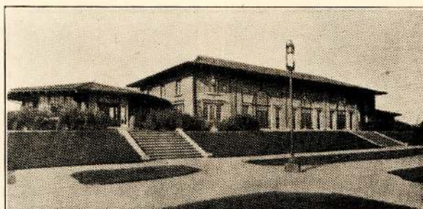
Recreation building and field house, South Parks, Chicago
