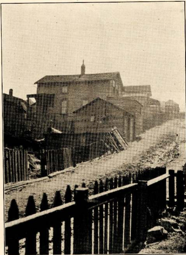
The building of houses in such locations as this should not be permitted
