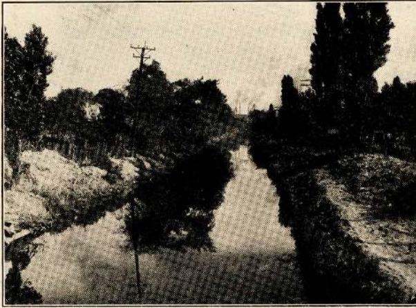
Park possibilities along the Ohio Canal, north from Thornton Street
