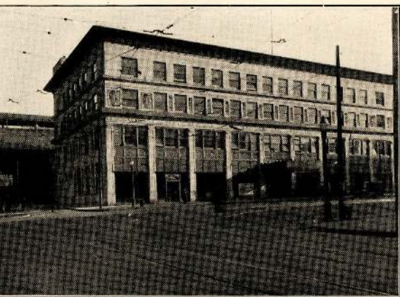
New Interurban Trolley Station at Akron, one of the most complete in the country
