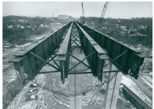
Construction of the Y-Bridge, 1980.
