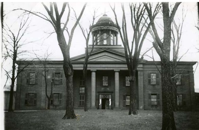
The Summit County courthouse about 1900. It was demolished in 1905 when construction of the present courthouse began. From the General Photograph Collection.
