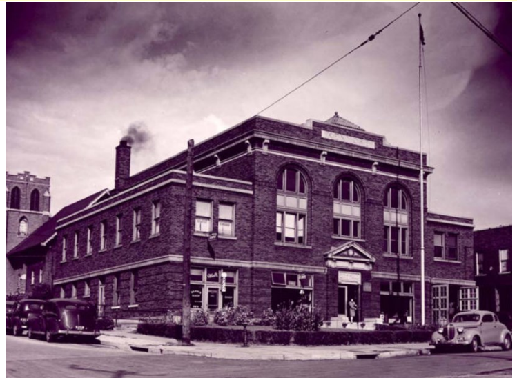
Kenmore City Hall about 1945. The Akron Public Library maintained a small branch on the second floor of the building from 1930 until the opening of the current branch location on Fourteenth Street SW in 1957. From the Library History Collection, Summit Memory.
