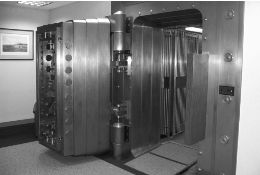
Figure 19 Safe deposit vault door.
