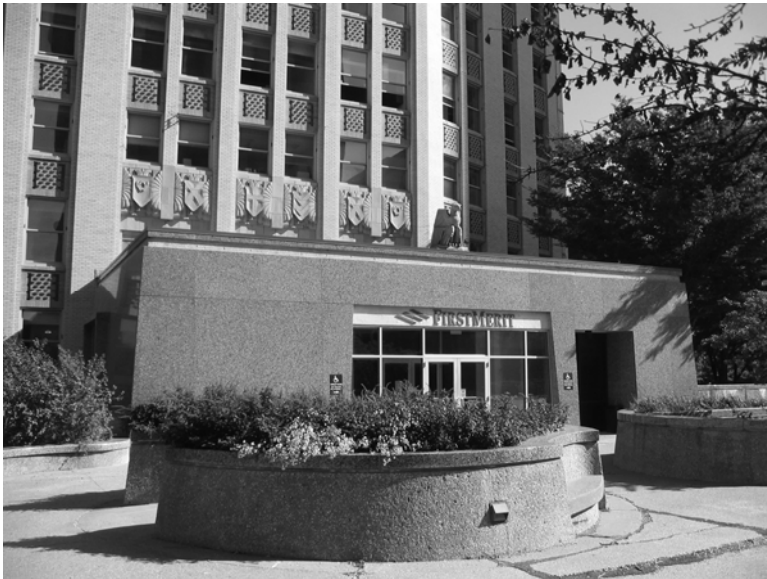
Figure 12 West entrance on to Cascade Plaza, 2005. This entrance, one level above the South Main Street level, replaces the Hower Street entrance that was eliminated with the parking deck and plaza construction in 1967.
