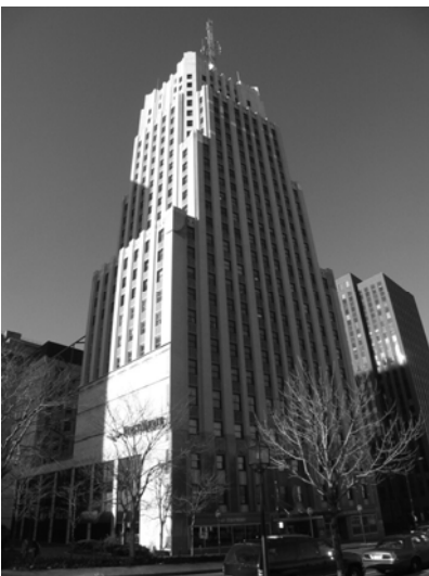
Figure 8 First National Bank from the southeast, 2005. Note the former party wall on the lower 6 stories of the south elevation, and the new banking hall windows inserted that wall.
