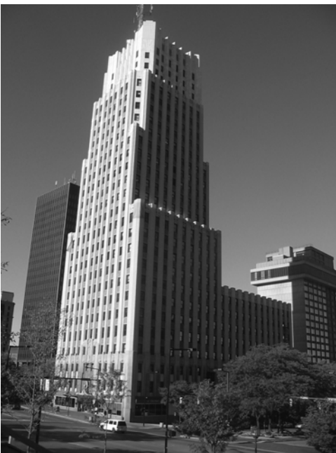
Figure 10 First National Bank from the northeast, 2005. Note the west annex to the right.
