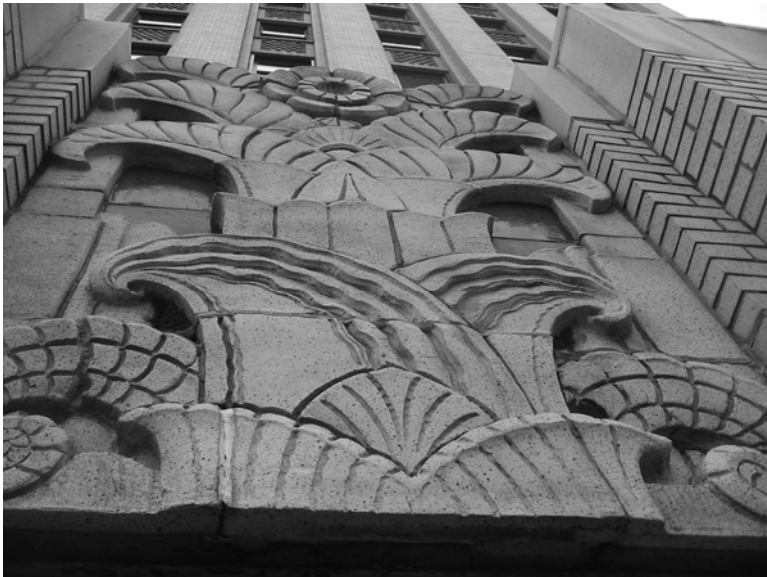
Figure 14 Typical decorative terra cotta parapet.
