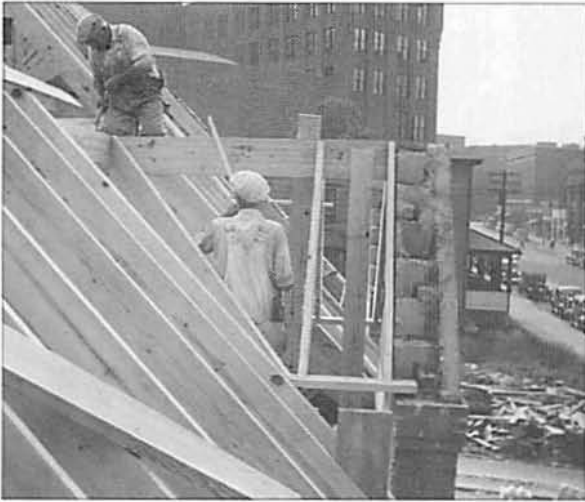
Workmen construct the roof of East Branch.
