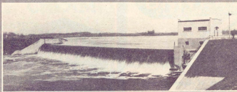
AKRON WATER WORKS DAM ACROSS CUYAHOGA RIVER.
