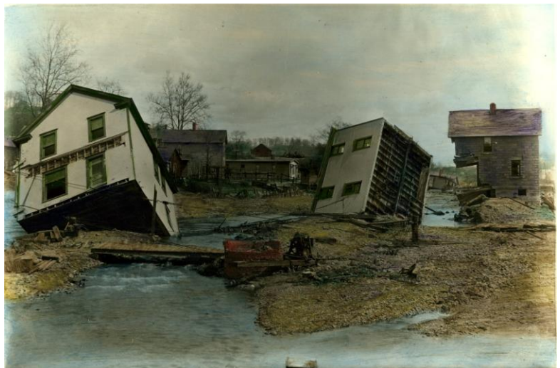
Buildings on East North Street wrecked by the Flood of 1913. From the Summit County Historical Society's Pockrandt Collection.
