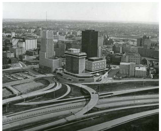
Aerial view of Cascade Plaza looking southeast after the demolition of South Howard Street. From Summit Memory.
