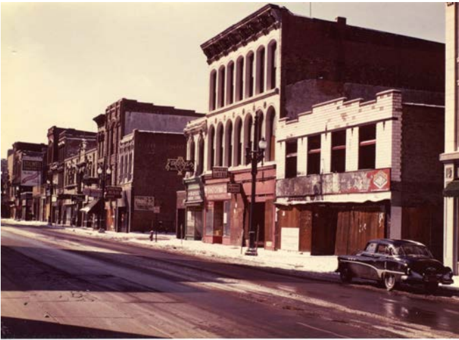
West side of South Howard Street before demolition. From the Cascade Plaza Urban Renewal Photographs collection.
