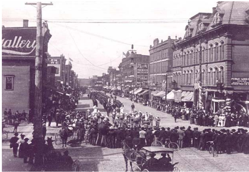
This photo of the 1897 Decoration (Memorial) Day parade in downtown Akron shows the Library's location in the former Masonic Temple building at the northeast corner of Mill and Howard (right center). From the Library History Collection.
