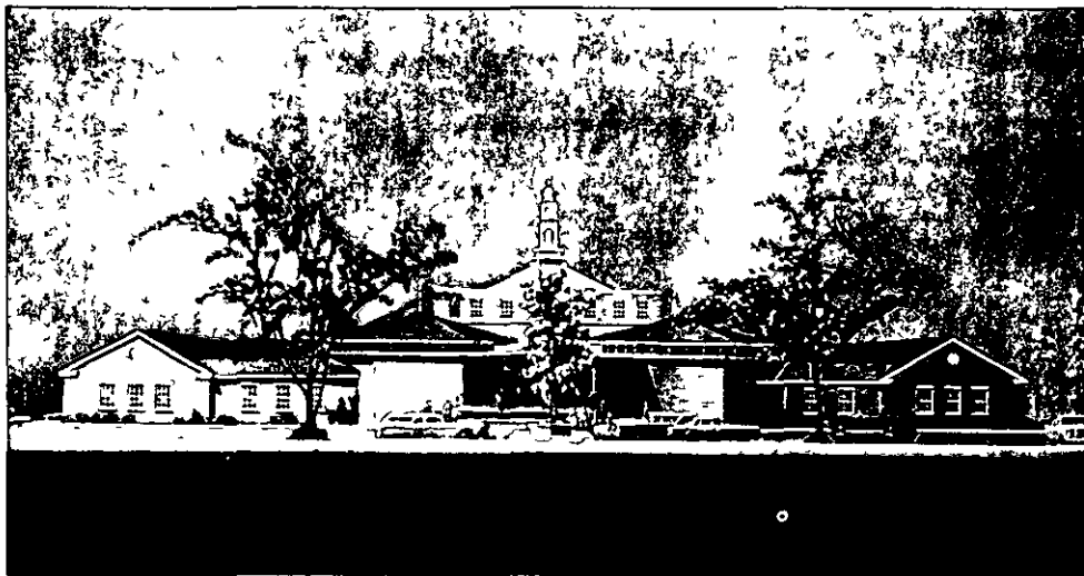
CUYAHOGA FALLS CITY BUILDING
